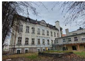
Forensic Psychiatry Facility in Branice
